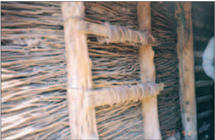
Willow, mud and log construction of barn on the Brace Ranch.
