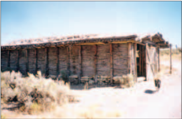
Barn at the Brace Ranch showing the unique construction. Made with double walls of willow switches packed between upright logs, reinforced with mud. Chuck Dougal built the doors and corrals when he and Frankie honeymooned and buckarooed there in the early 1930s.
